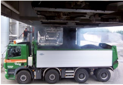
Asphalt and concrete mixing
