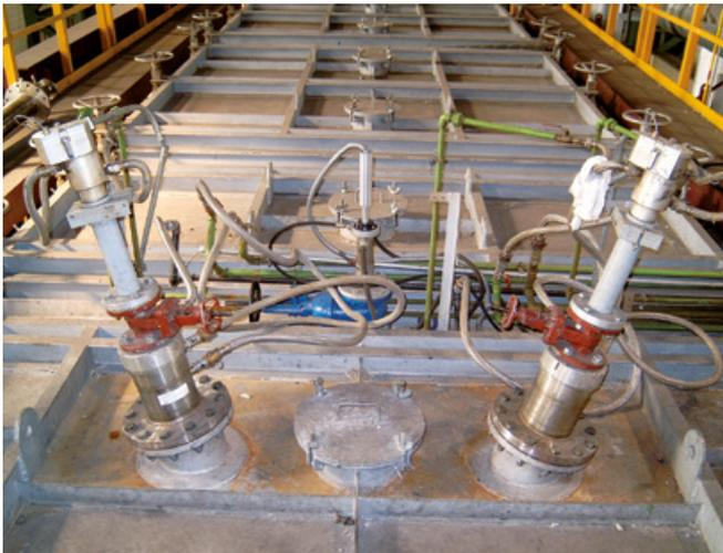
**Picture 7** Though measuring the same target, the devices showed large temperature differences due to wrong focal adjustment.
