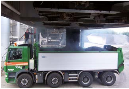
Asphalt and concrete mixing
