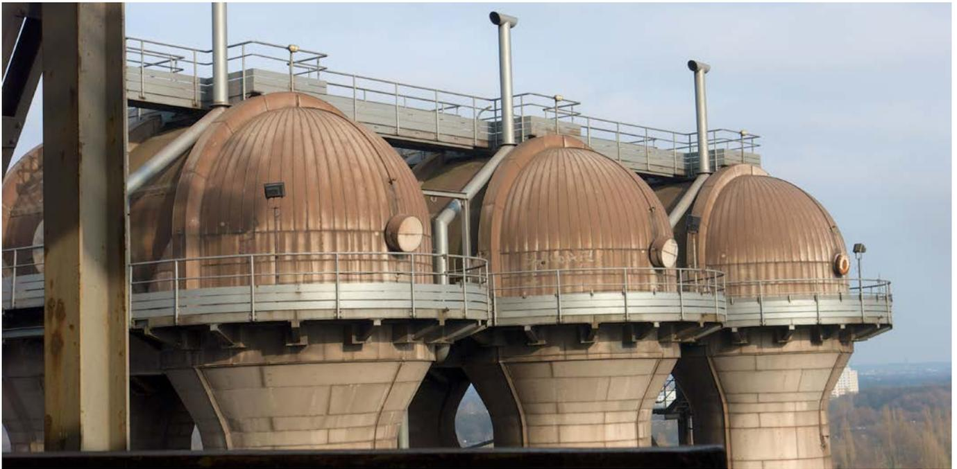
**Fig. 1** Pyrometers measure the temperature of the checker bricks in the stove dome from the cupola.
