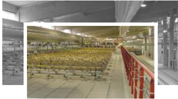
Top fired tunnel kiln
